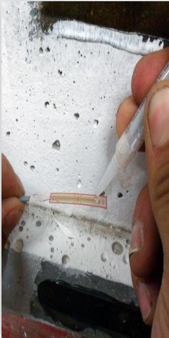
Applying CN-E adhesive
