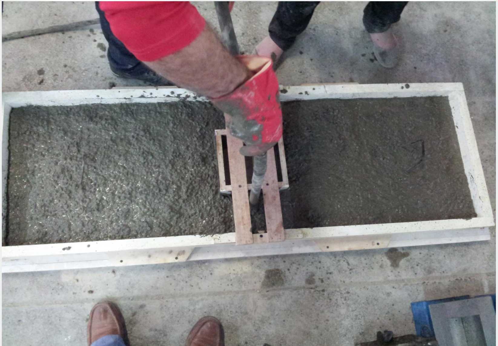
Figure (1 v ) Compacting with Rod Vibrator
