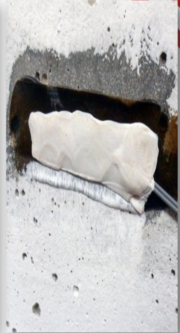
Coating with SB tape
