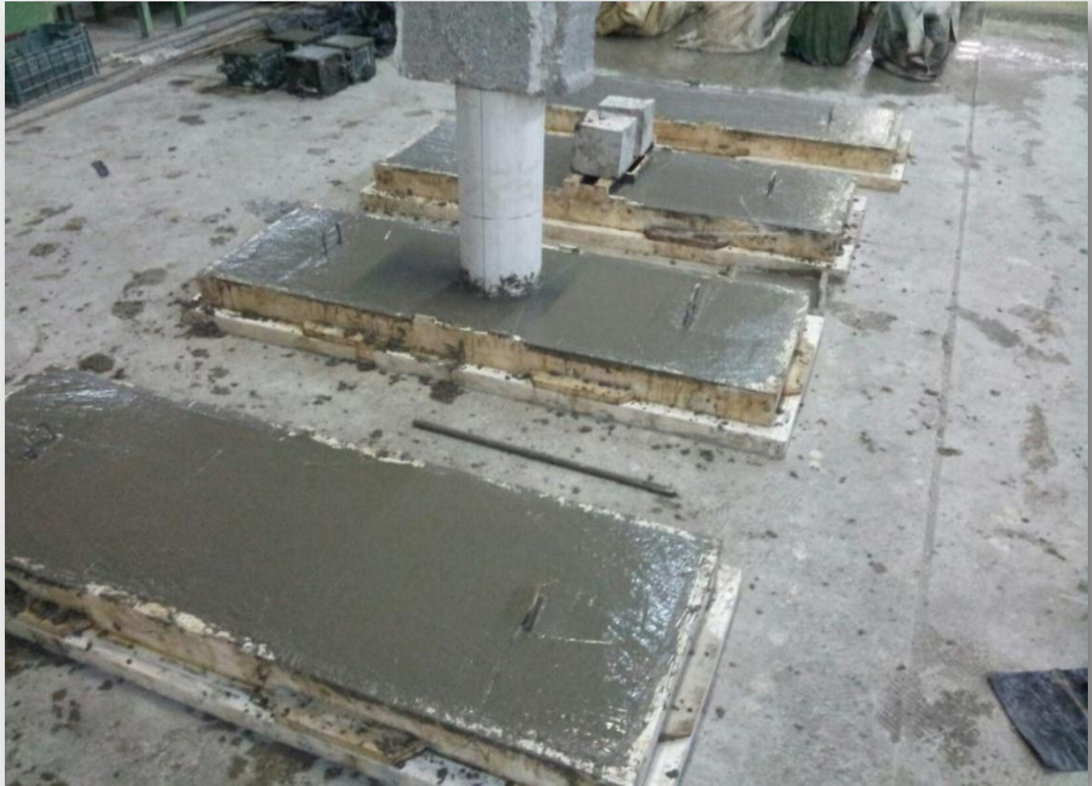
Figure (1 o ) Concrete Mixing and Placing
