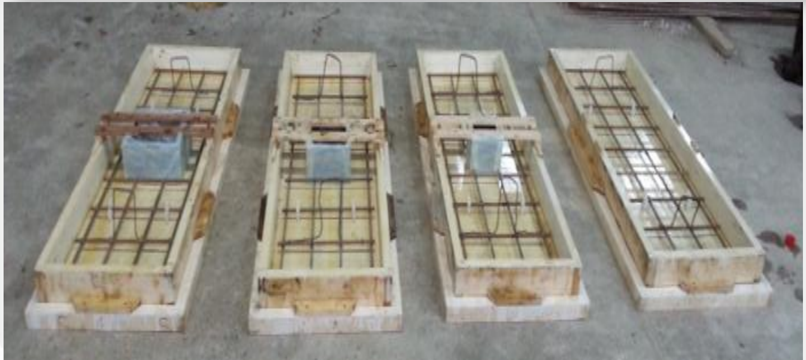
Figure (9) Preparing Wooden Molds for Slabs and Openings.
